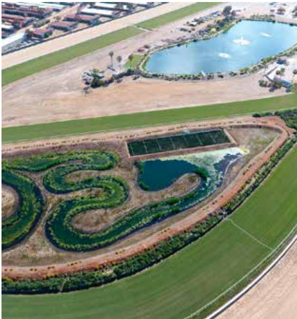
Del Mar Fairgrounds Infield Water Quality Project
