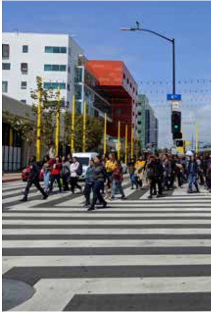
Enhanced crosswalk markings
