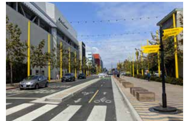
Class IV separated bikeway
