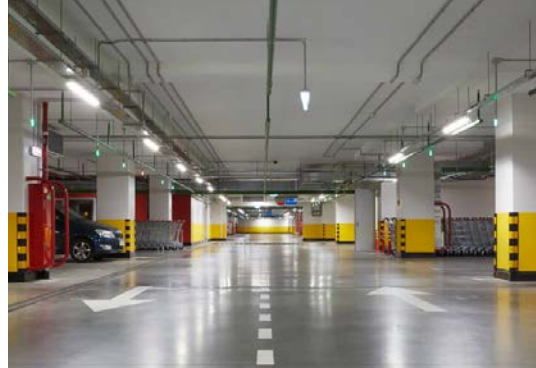
Stand-alone parking structure
