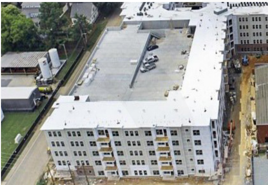
Structured parking wrapped with residential as part of a mixed-use development
