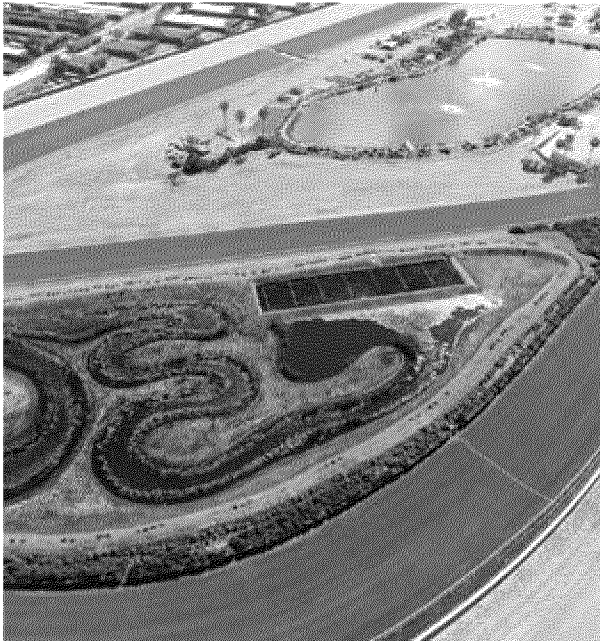
Del Mar Fairgrounds Infield Water Quality Project
